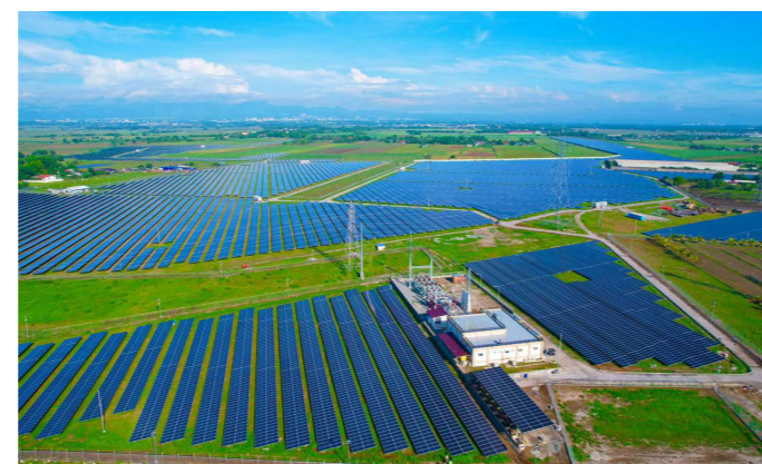
The 72 MW first phase of the Arayat-Mexico Solar Farm, a joint venture between ACEN and Citicore, started operations in 2022. It is expected to generate 105 GWh of renewable energy annually, which can power approximately 45,000 homes.
