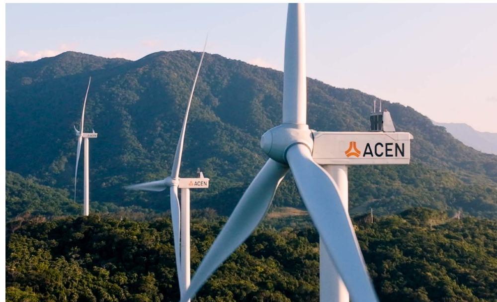
The 160 MW Pagudpud Wind in Ilocos Norte comprises 32 wind turbine generators, each capable of producing 5 MW of power.
