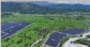
SanMar Solar (Phase 3) 200 MW dc San Marcelino, Zambales
