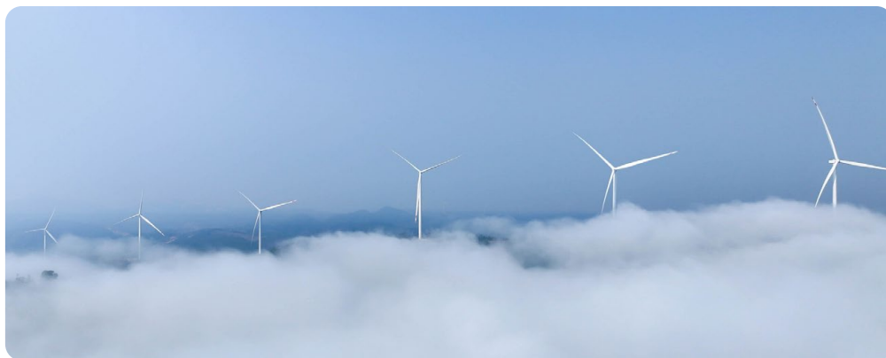
In 2025, the 600 MW Monsoon Wind project was delivered ahead of schedule and within budget, overcoming complex, multi-stakeholder coordination during construction.
