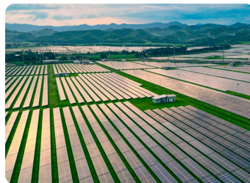
To restore plant efficiency and enhance energy output, our 45 MW SaCaSol in Negros Occidental is replacing select solar panels, with the works scheduled for completion by 2026.
