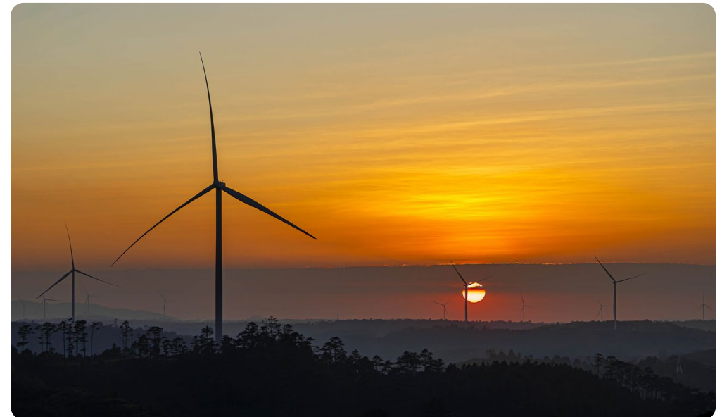
Stretching across Lao PDR’s Dak Cheung District of Sekong Province and the Sanxay District of Attapeu Province, 133 wind turbines of the 600 MW Monsoon Wind rise from the ridgelines, turning steadily in the region’s strong, reliable winds.
