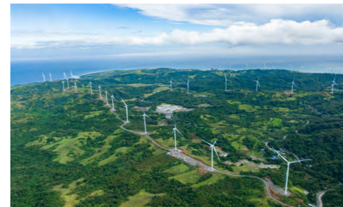
Located in Barangays Balaoi and Caunayan across Pagudpud town in Ilocos Norte, ACEN's 160 MW Pagudpud Wind comprises of 32 wind turbine generators, each capable of producing 5 MW of power to optimize production of renewable energy.
