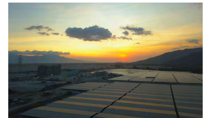
The first and second phases of our 585 MW SanMar Solar already began injecting power to the grid in December 2023 as part of its testing and commissioning program. With the third phase's construction in full swing, SanMar Solar's expansion reinforces our mission to supply more renewable energy to the Philippines' energy grid.
