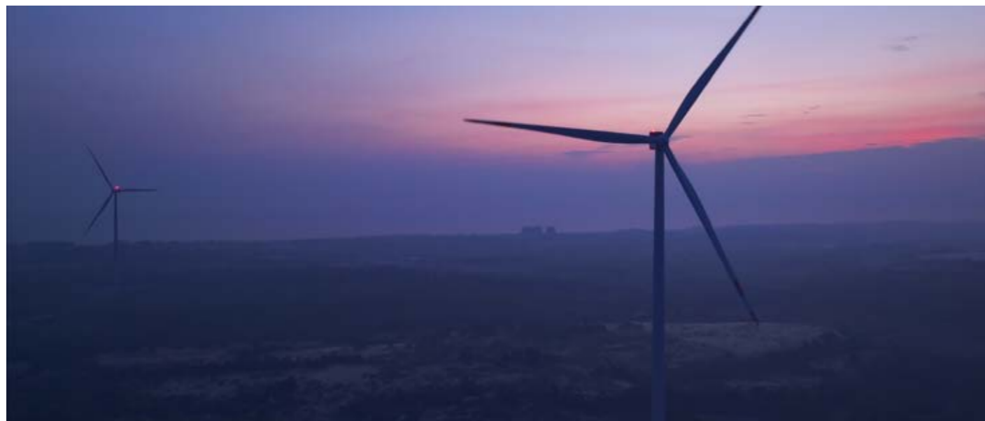
The 252 MW Quang Binh Wind, a project we co-developed with AMI, significantly contributes to Vietnam's clean energy and climate action targets and is instrumental to our massive renewables expansion in the region.
