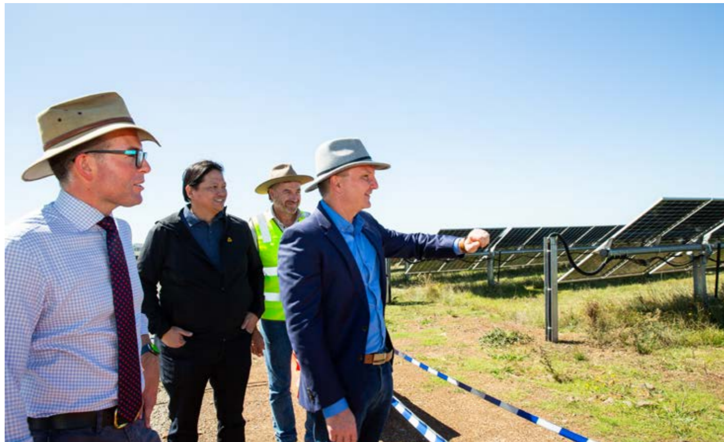
One of Australia's largest solar projects, the first stage of ACEN's 521 MW New England Solar was officially opened in March 2023 by Australia's federal minister for climate change, Hon. Chris Bowen MP.
