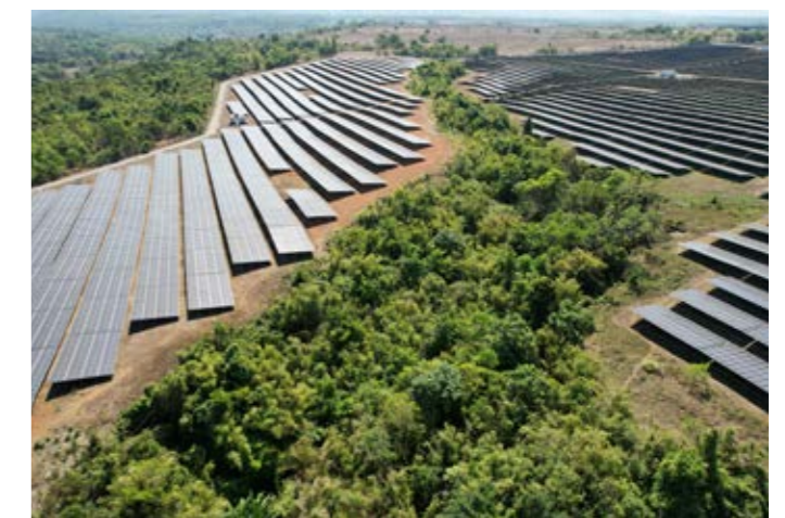
Our 63 MW Palauig Solar 1's energy consumption initiatives are an example of how we are championing resource efficiency in our operations.
