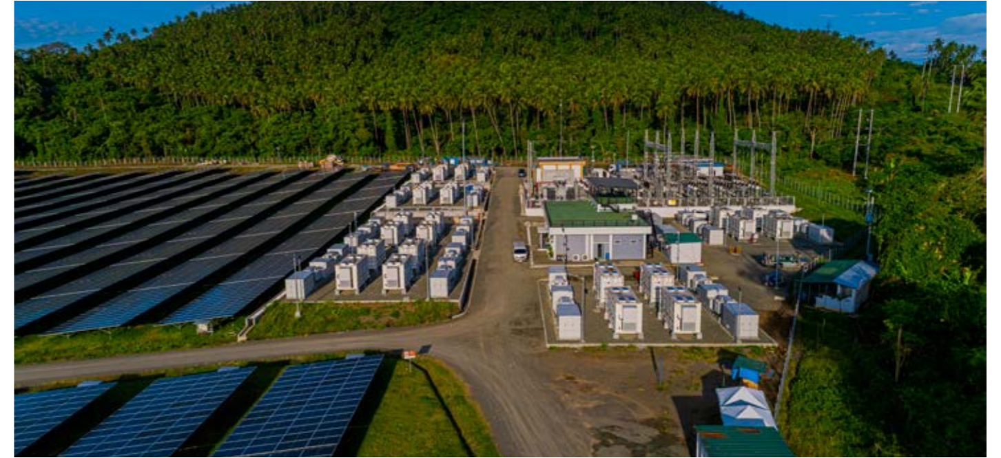
During the early development phase of our 120 MW Alaminos Solar in Laguna, Philippines, we integrated a plastic recycling facility to collect plastic waste and upcycle them into eco-bricks, which were used in building the solar plant facilities.
