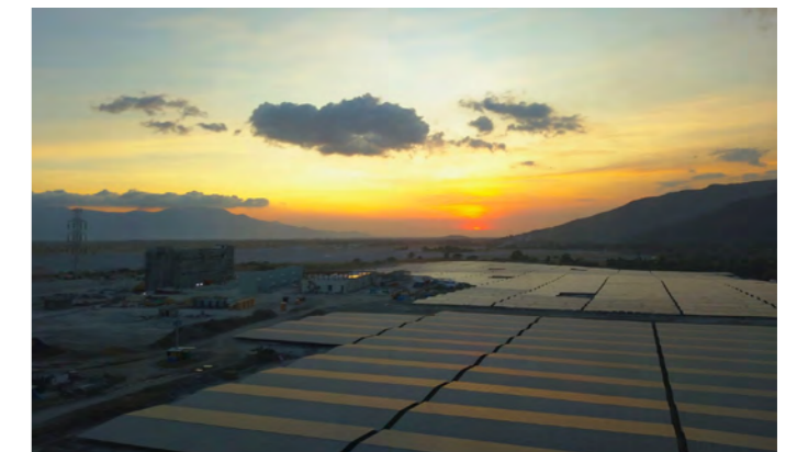
The first and second phases of our 585 MW SanMar Solar already began injecting power to the grid in December 2023 as part of its testing and commissioning program. With the third phase's construction in full swing, SanMar Solar's expansion reinforces our mission to supply more renewable energy to the Philippines' energy grid.
