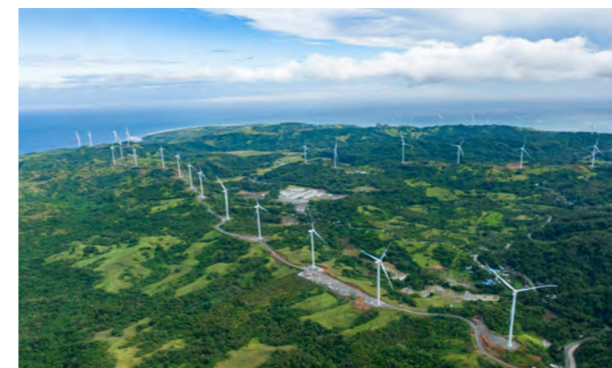
Located in Barangays Balaoi and Caunayan across Pagudpud town in Ilocos Norte, ACEN's 160 MW Pagudpud Wind comprises of 32 wind turbine generators, each capable of producing 5 MW of power to optimize production of renewable energy.
