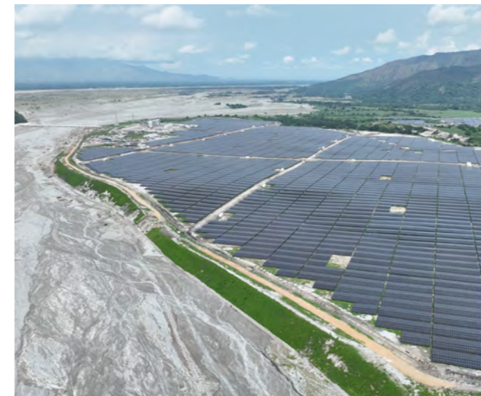
In San Marcelino, Zambales, our 585 MW SanMar Solar, which sits on over 500 hectares of idle land covered by lahar, is touted as the largest solar farm in the Philippines to date. Its third phase is expected to finish construction by 2025.
