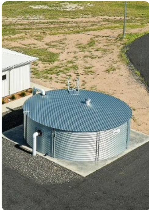
The rainwater harvesting tank at Stubbo Solar in Australia.
