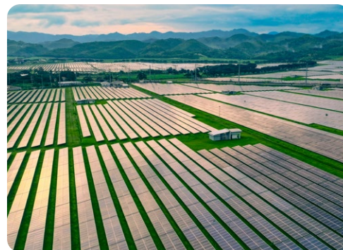
To restore plant efficiency and enhance energy output, our 45 MW SaCaSol in Negros Occidental is replacing select solar panels, with the works scheduled for completion by 2026.
