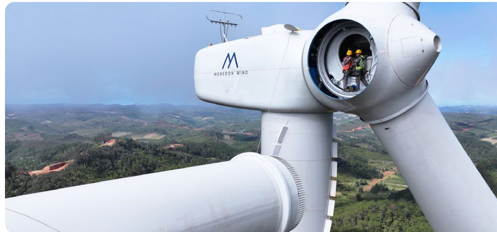
600 MW Monsoon Wind, the first cross-border wind farm located in Lao PDR, delivers clean electricity to Vietnam.
